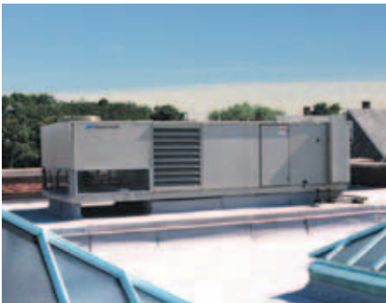
Replacement Rooftop Systems
