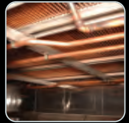
Evaporative-cooled condensers with chemical free water treatment
