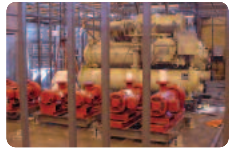
Packaged chiller plants save design and installation time and costs.
